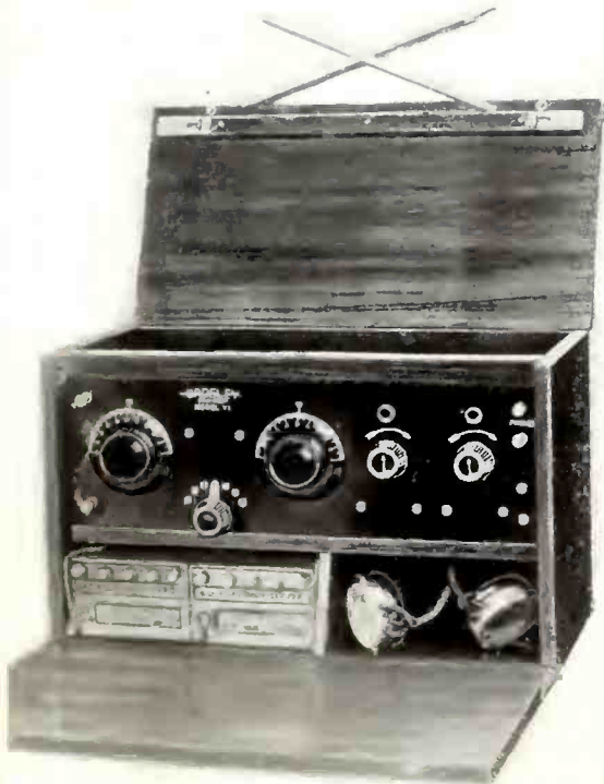
Two-tube Crosley model VI had RF and detector. Two 22½-volt "B" units.
